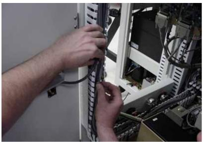
Figure 1-13—Route wire harness into cable guide #1
