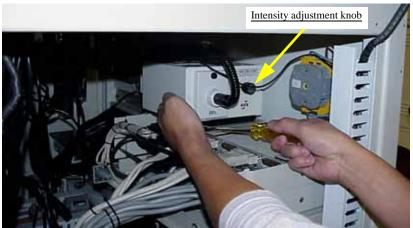
Figure 1-21—Light source with intensity adjustment knob visible
