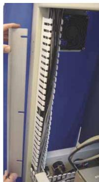
Figure 1-12—Slide door support between frame and cable guide #1
