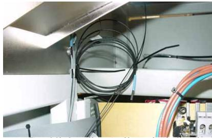
Figure 1-10—Secure fiber optic cables to underside of base plate
