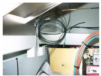
Figure 1-45—Secure fiber optic cable to underside of base plate
